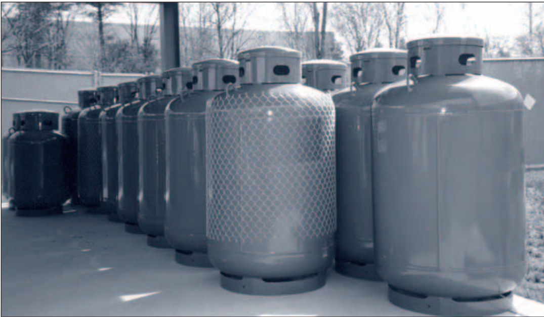
FIGURE 8-13 100 gallon (420 lb.) propane tanks.
